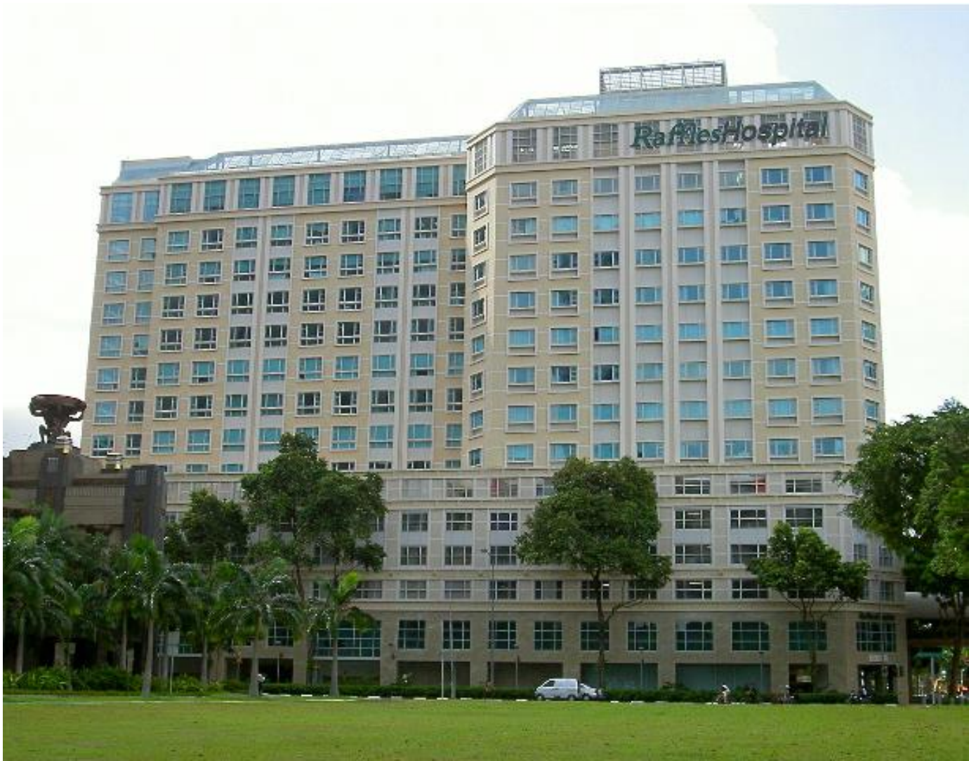
Curtain & Sunscreen at Raffle Hospital - Singapore
